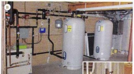
What goes up must come down: The wind turbine will be dropped every five years for general maintenance and lubrication (A). In the basement, an Econar ground-source heat pump uses the drinking well to provide
