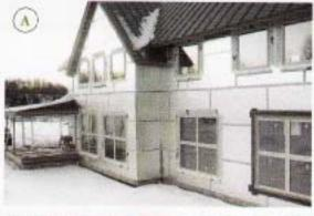
An exterior skin of foil-faced polyiso — with seams taped and windows tightly flashed — helps seal the shell and further reduces thermal bridging (A). Pre-drywall blower-door testing (B) done in conjunction with an infrared camera (C) helped to locate air leaks in the tightly insulated interior (D).
