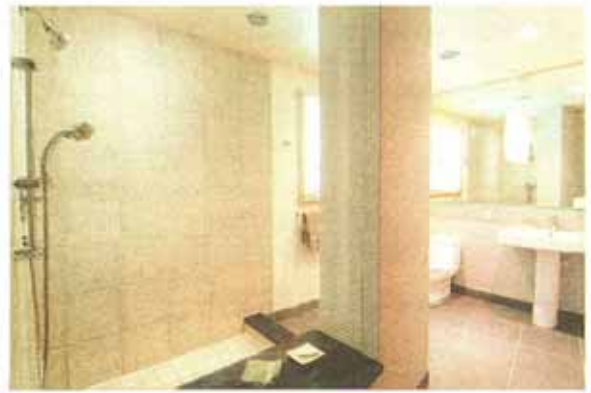
THE MASTER BATH was carved into a space in the house that was originally a child's bedroom. The bathroom now connects to the master bedroom via a dressing room/closet. The oversized tiled shower is separated from the dressing area by a glass divide that sits atop a slate bench. The floor and walls are finished in ceramic tile.
