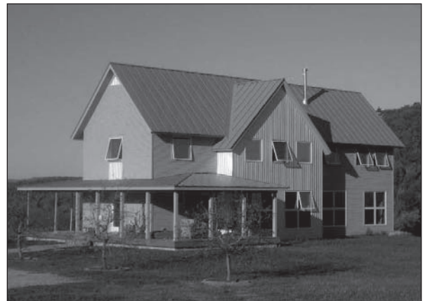
Figure 4. Most of the Pill house’s windows face south. The siding is a mixture of white-cedar clapboard and Galvalume metal siding.
