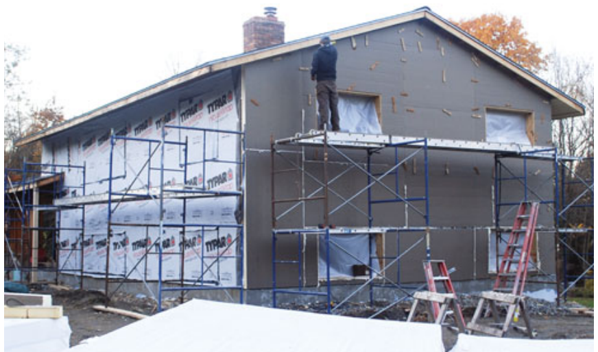
Figure 2. After removing the old windows and installing plywood window bucks, workers wrapped the walls with 4x8 panels of 4-inch-thick polyisocyanurate foam (top). The panels were glued to the vertical cedar siding, and plywood cleats secured with long screws were used to temporarily hold them in place until the glue set (center and above).
