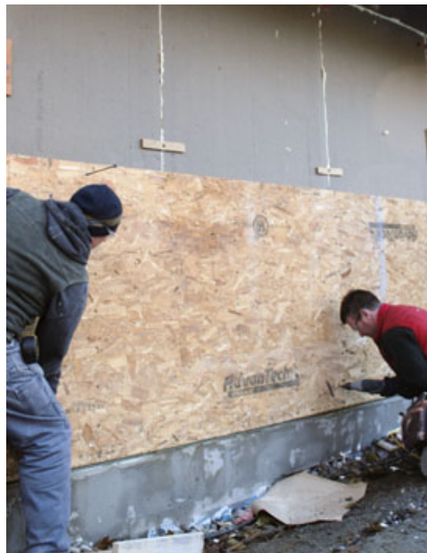
Figure 4. The tongue-and-groove profile along the edges and the biscuits at the butt joints (far left) kept the panel edges flat. Since the panel ends were biscuited together, the panels didn't have to be trimmed to fit the stud layout (left). An intentional \frac{3}{4} -inch gap was left between the insulation-sheathing assembly and the foundation insulation and later filled with spray foam (above).
