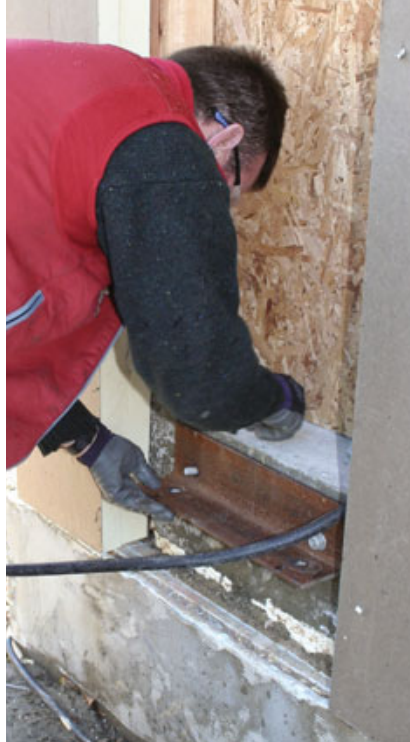
Figure 5. Sections of 3\frac{1}{4} -inch by 3\frac{1}{4} -inch by \frac{1}{4} -inch steel angle were bolted to the wall underneath the door openings (left and above). The angles were then padded with PT blocks and shims until the door sills were fully supported (illustration, below).
