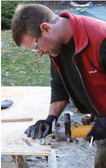
Figure 3. Before installing the AdvanTech sheathing, the carpenters cut slots for biscuit joints in the butt ends of the panels (left) and predrilled countersunk holes for the structural screws (above left). The sheathing was also glued to the foam panels with a low-VOC construction adhesive (above right).
