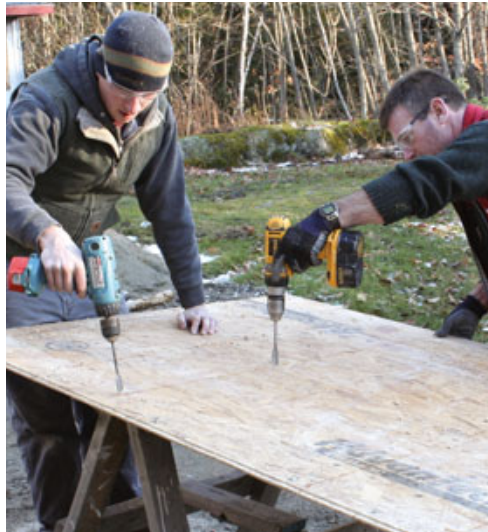
Figure 3. Before installing the AdvanTech sheathing, the carpenters cut slots for biscuit joints in the butt ends of the panels (left) and predrilled countersunk holes for the structural screws (above left). The sheathing was also glued to the foam panels with a low-VOC construction adhesive (above right).
